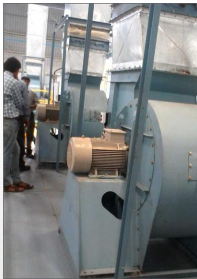
Application - Top Coat Booth Customer - SAPL, Chakan FAN - 30HP
