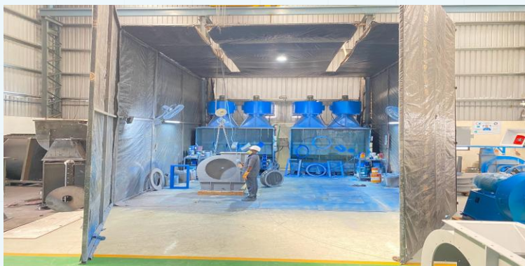
Blast & paint — DFT checked at every stage
